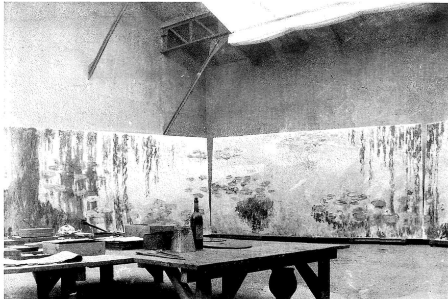
101. Interior of the third studio before a ventilator was installed in the southeast corner in late April 1916.
