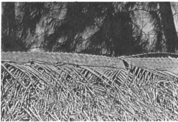
80. Rooftop of plaited coconut palm leaves.
